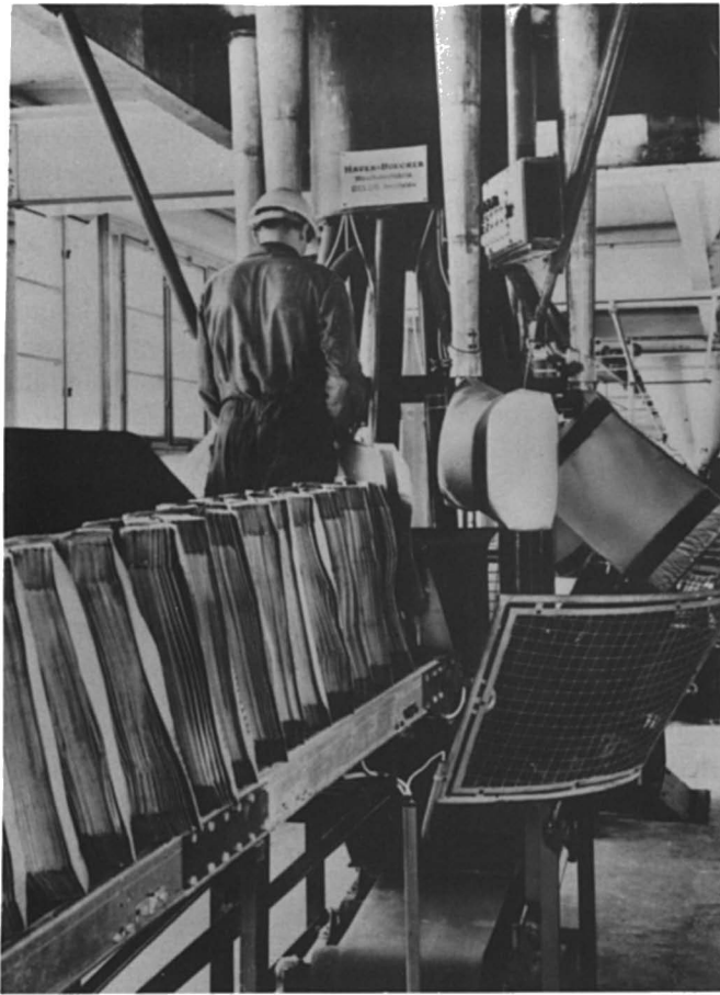
Photo 3 Filling Valve Bags Using The Free-Fall Roto Packer
