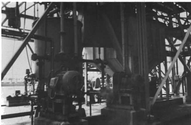
Slide 4 REACTOR SLURRY TANK AND PUMPS
