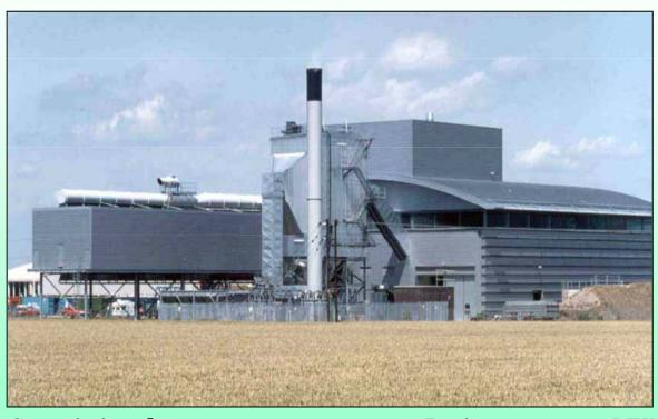
Commissioned 1992 Design output 12.7 MW Burns 170,000 ton/yr. of poultry litter & other biomass
