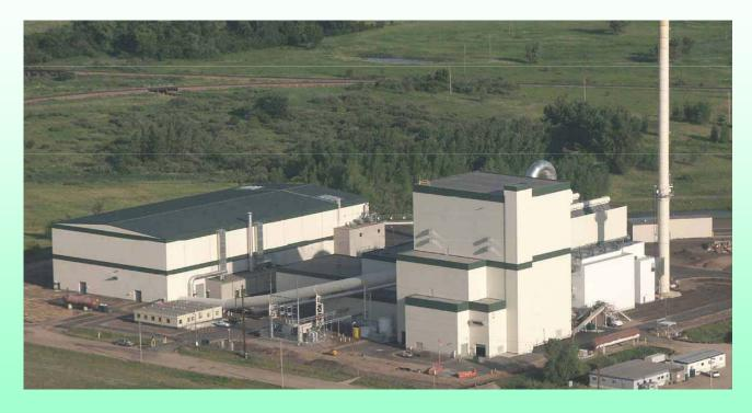
Commissioned October 2007 Design output 55MW Will combust over 700,000 ton/yr. of poultry litter & other biomass
