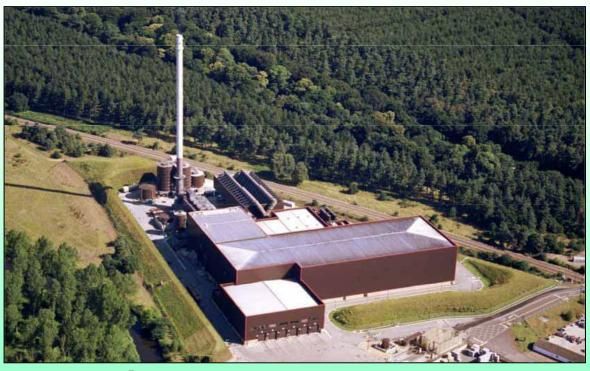
Commissioned 1998 Design output 38.5MW Burns 500,000 ton/yr. of poultry litter & other biomass
